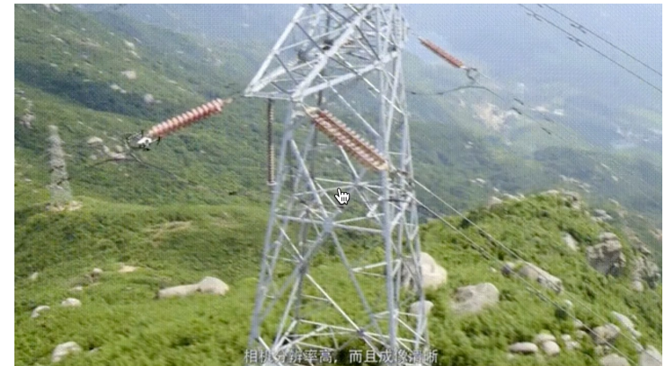
Drones surveying a high-voltage system in Guilin
