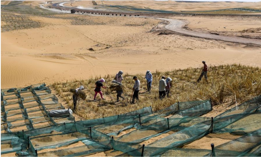
Desertification control workers make straw checkerboard barriers in the Tengger Desert along the construction site of the Qingtongxia-Zhongwei section of the Wuhai-Maquin highway in northwest China's Ningxia Hui Autonomous Region, Sept. 7, 2020. (Xinhua/Feng Kaihua)
